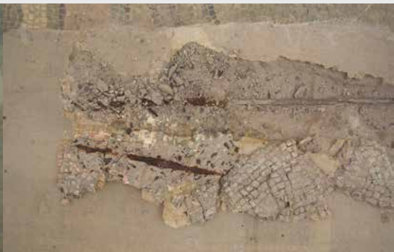
Reinforced iron bars removal
