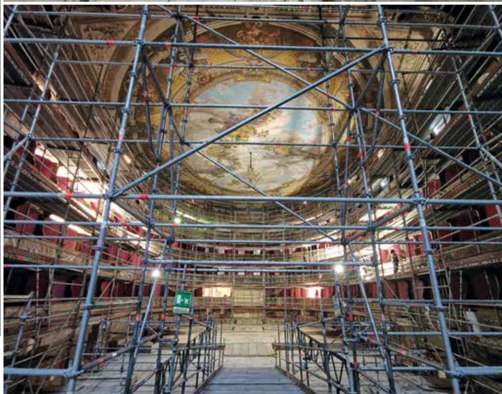
The main hall and its decorated ceiling during the restoration
