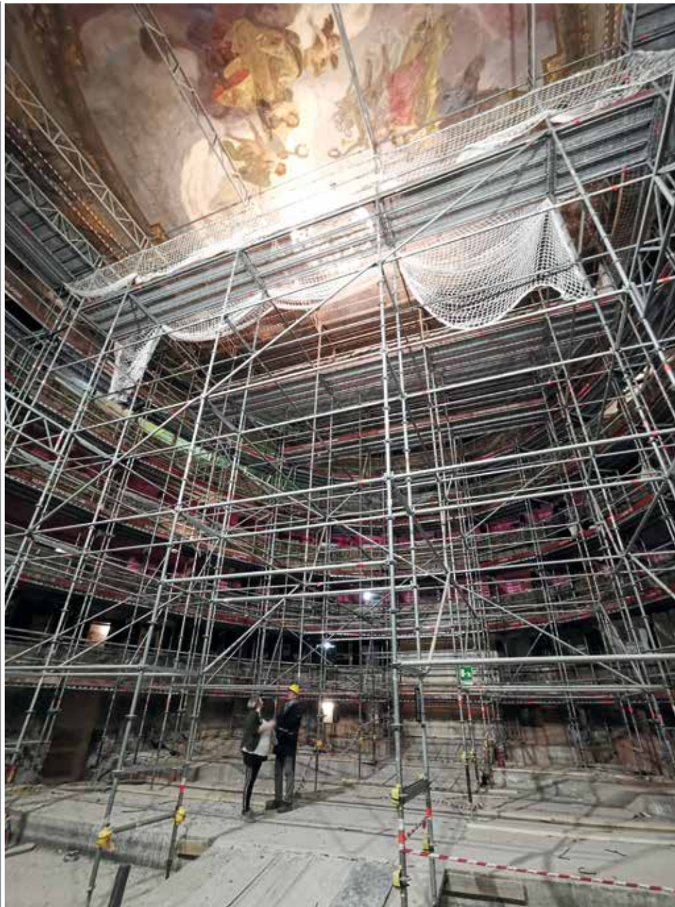
The main hall of the Theatre during the interventions
