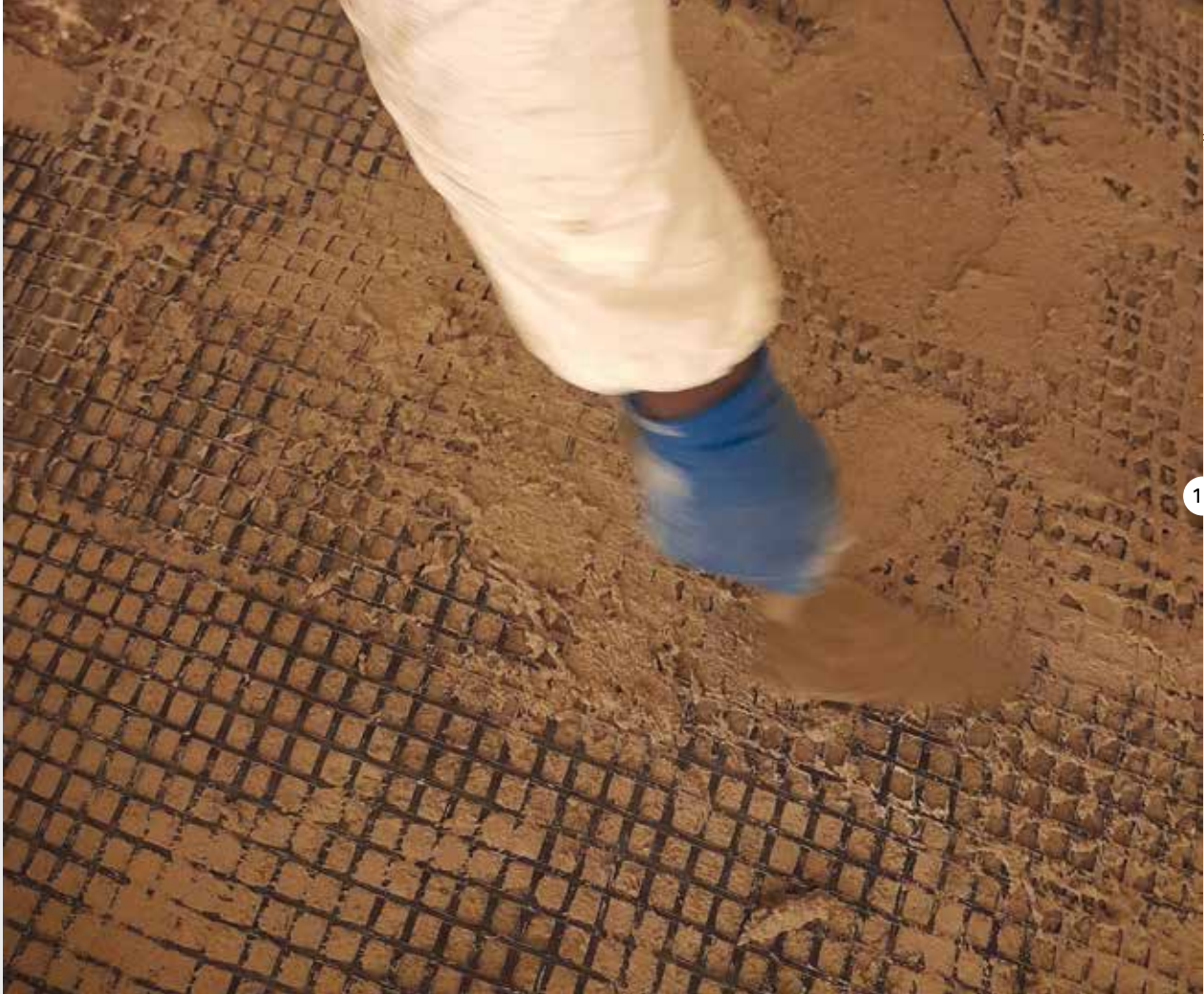
Fig 8. Reinforcement of arched vaults with GFRP
