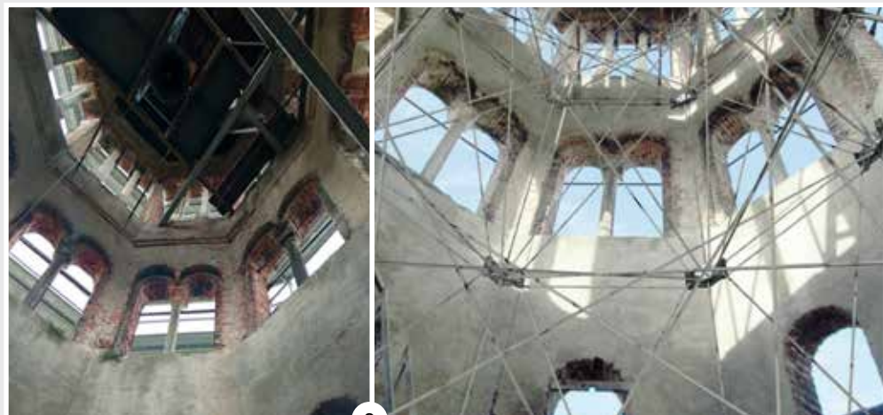
Fig 3. Final configuration of the structural reinforcement
