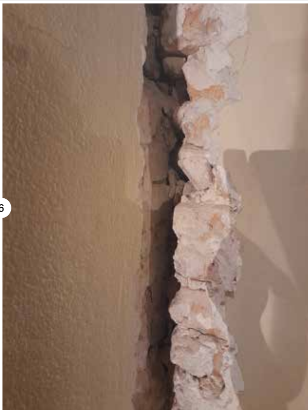
Fig 7. Stitching with stainless steel elements inserted in the restyling of flat lesions
