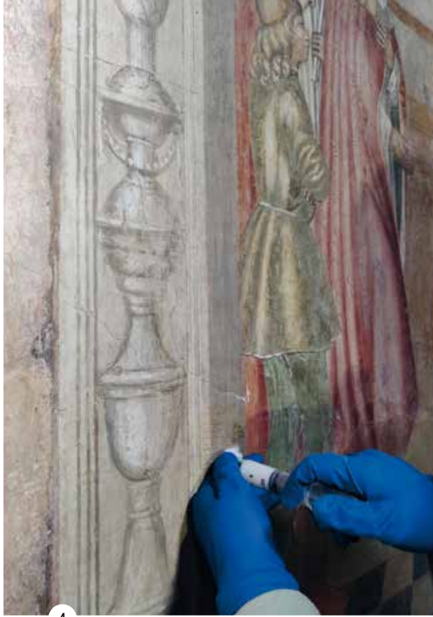
Fig 4. Plaster consolidation of the Pio's Chapel by Cooperativa Archeologia's team of experts
