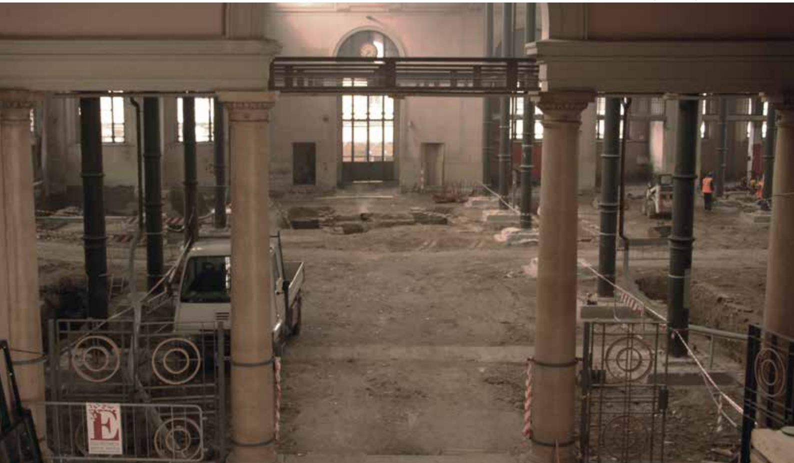
Panning from the top of the excavation yard
