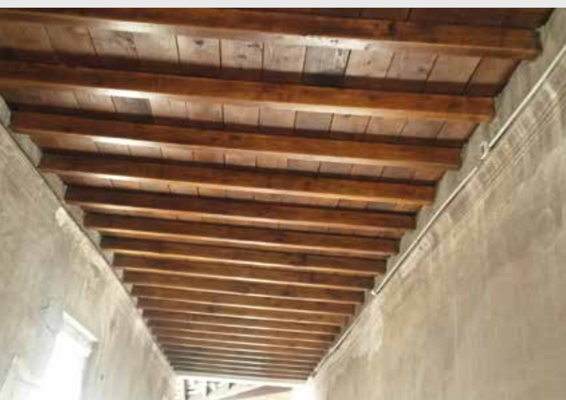
Attic floor wooden
