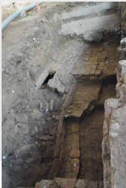
Coverage of the river Padenna of the XV century. Seen by South. We clearly seen as the vault has been used as support for the construction of building and floor structures of following epochs.
