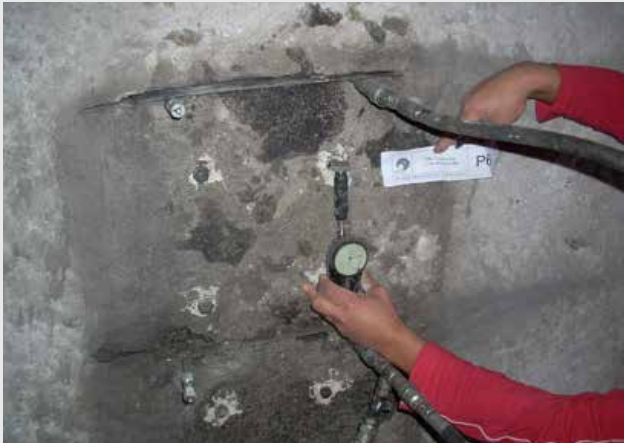
On-site test with Double Flat Jacks
