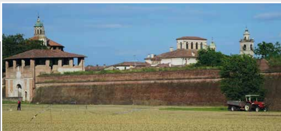
The city walls of Sabbioneta: present state and situation in 1985. The walls were built within 3 campaigns (1556-67, 1578-79, 1584-1600) in the shape of an irregular hexagon. They were abandoned for centuries and restored since 1994 (Photo D. Del Curto/Private collection)
