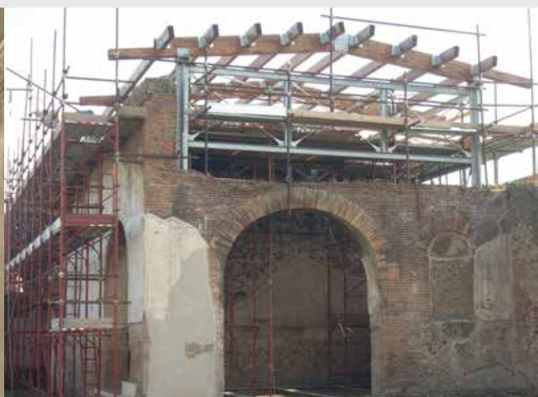
Restoration with full cover bering structure walls
