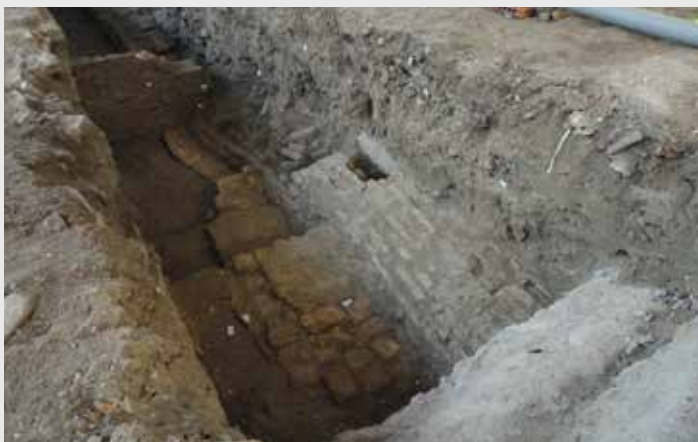
Coverage of the river Padenna of the XV century. Seen by South. We clearly seen as the vault has been used as support for the construction of building and floor structures of following epochs.
