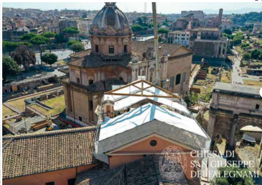
Fig 03. Photograph of the construction site from above
