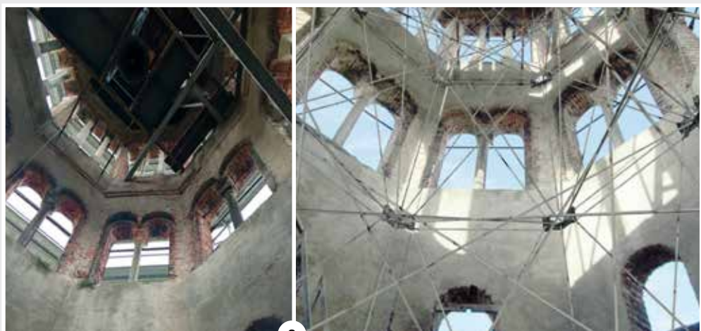
Fig 3. Final configuration of the structural reinforcement
