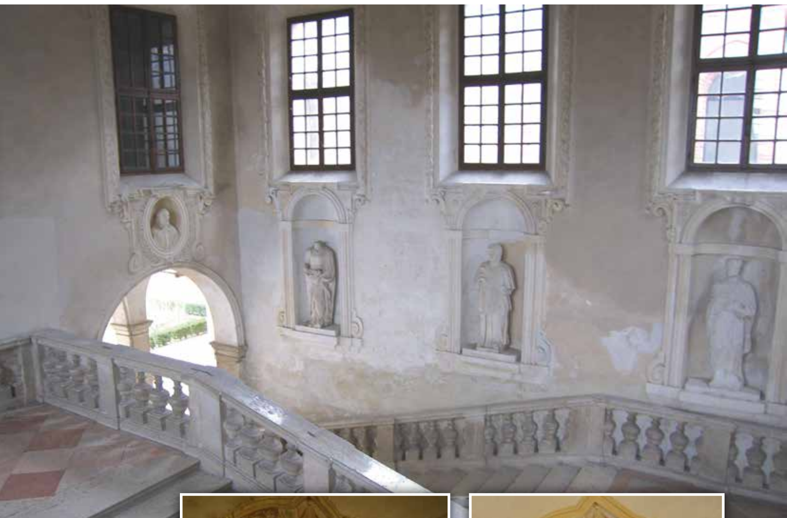
The monumental stairway before and after the restoration
