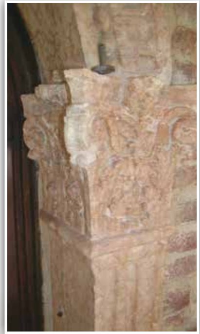
Juliet's house, frame with Corinthian capitals after the restoration
