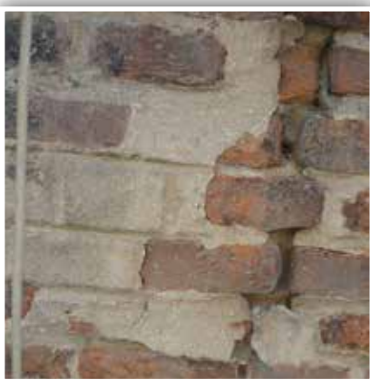
Figure 3. Juliet's house, facade, fragments of ancient plaster, made of a grout of lime and sand
