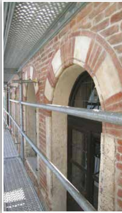
Figure 10. Juliet's house, facade after the cleaning and consolidation
