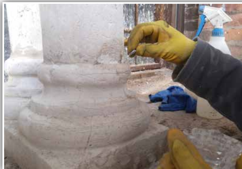
Grouting of pilaster fissures
