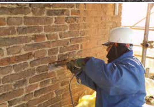
Removal of damaged bricks
