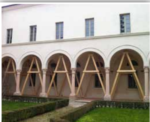
The provisional reinforcement of the arches in the "Secolari" cloister
