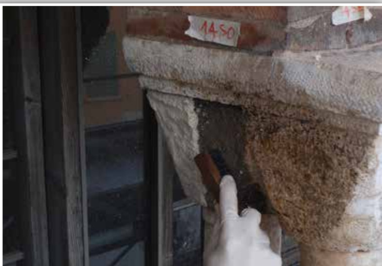
Preliminary surfaces cleaning
