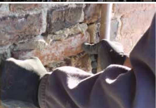
Replace of bricks
