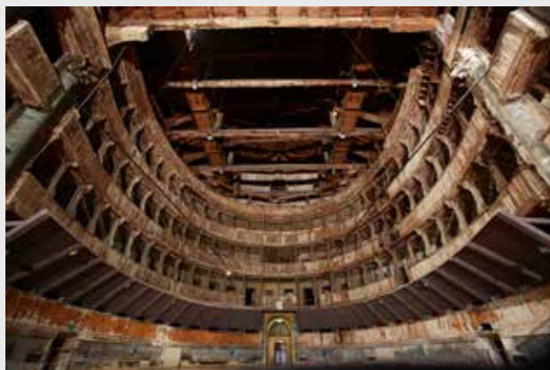
The main hall of the theater and the wooden parapeet of the boxes before the beginning of the restoration. The advanced state of degradation can easily be noticed.
