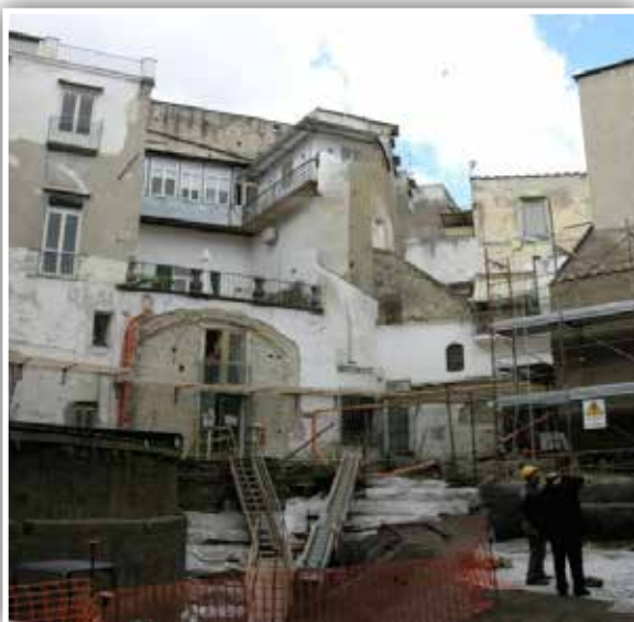
The emergence of the cavea after the excavation of the garden
