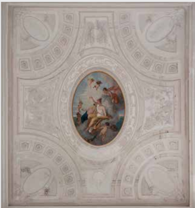
Ceiling before restoration
