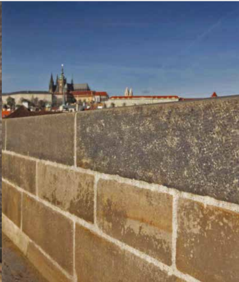
A detail view of the bridge after completion of the repairs
