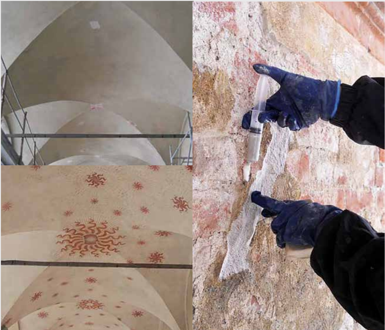
vault Rocchetta 's courtyards before and after restoration
