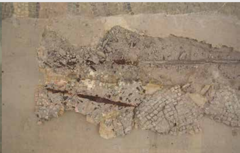
Reinforced iron bars removal
