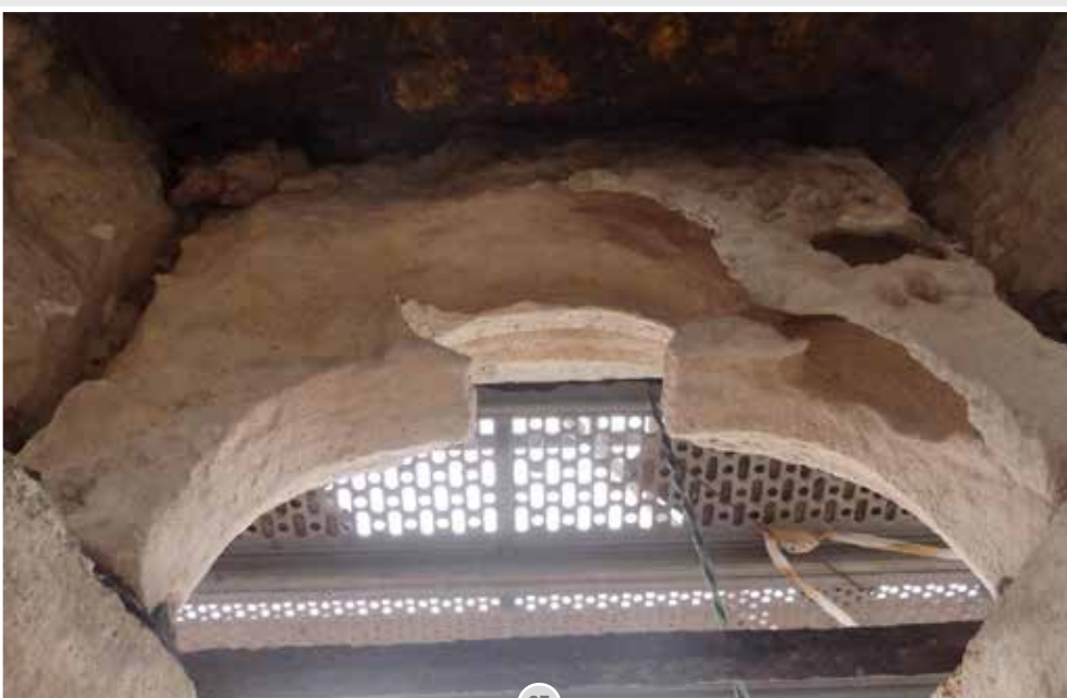
Fig 5-6. Details, erosion, Pinnacle of the Southern Transept
