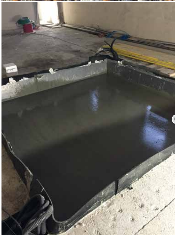
Fig 6. Casting of Betonfix CR pourable mortar
