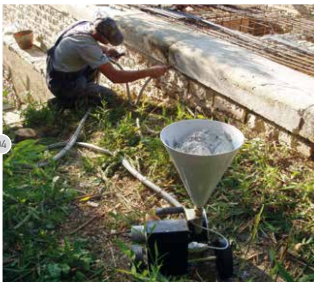
Fig 3-4-5. Sealing of joints
