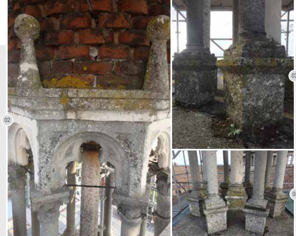
Fig 2-3-4. Details, biological degradation, Pinnacle of Southern Transept
