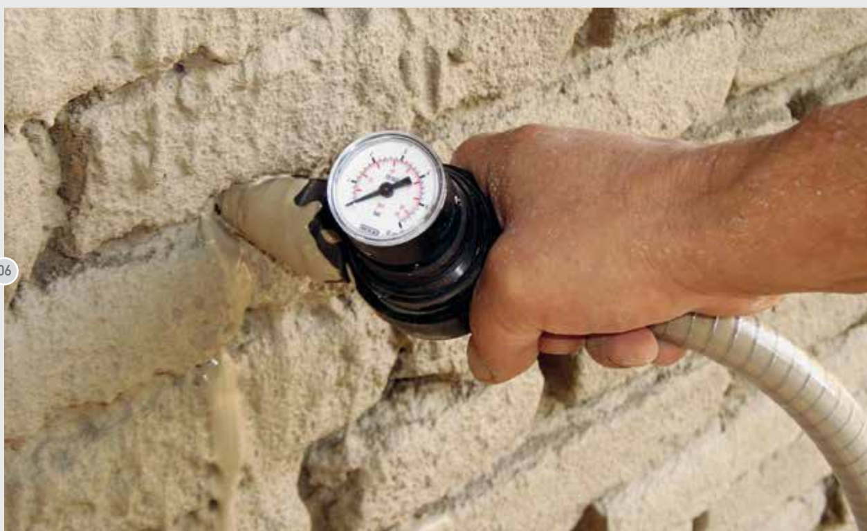
Fig 7-8. Microinjection version
