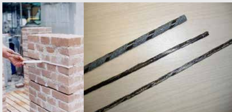
Reinforced repointing using FRP rebars
