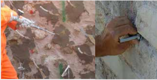
Multi leaves stone masonry injection and transversal tying
