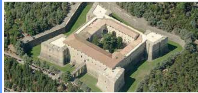
Spanish Fortress severely damaged by the 2009 earthquake
