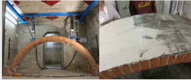
Vaults strengthening by using natural/artificial fibers and lime mortars
