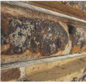
Example of steel ties connecting intersecting walls
