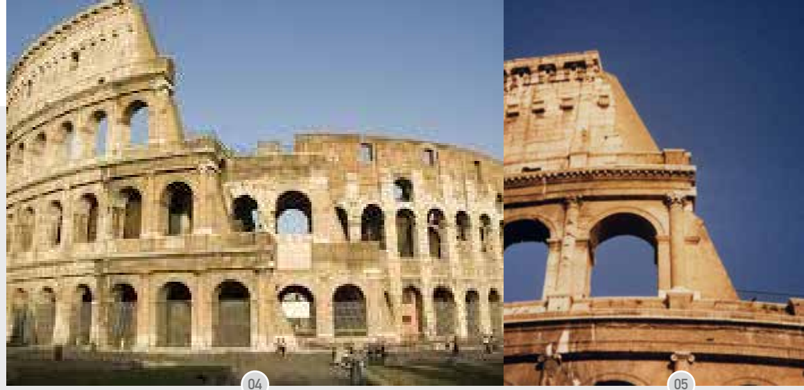
Fig. 04-05 Rome, Colosseo: Consolidation made by G. Valadier (1823)
