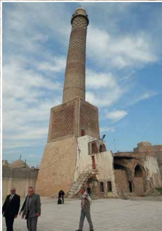
Fig. 25 Pictures of the Al-Hadba Minaret of the Mosque of Mosul and the consolidation project
